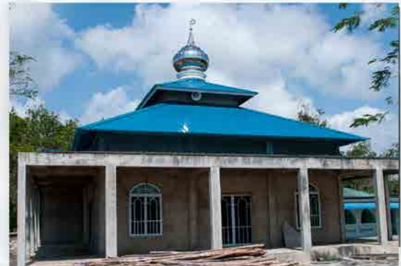
Renovasi Masjid Renovation of Mosque
